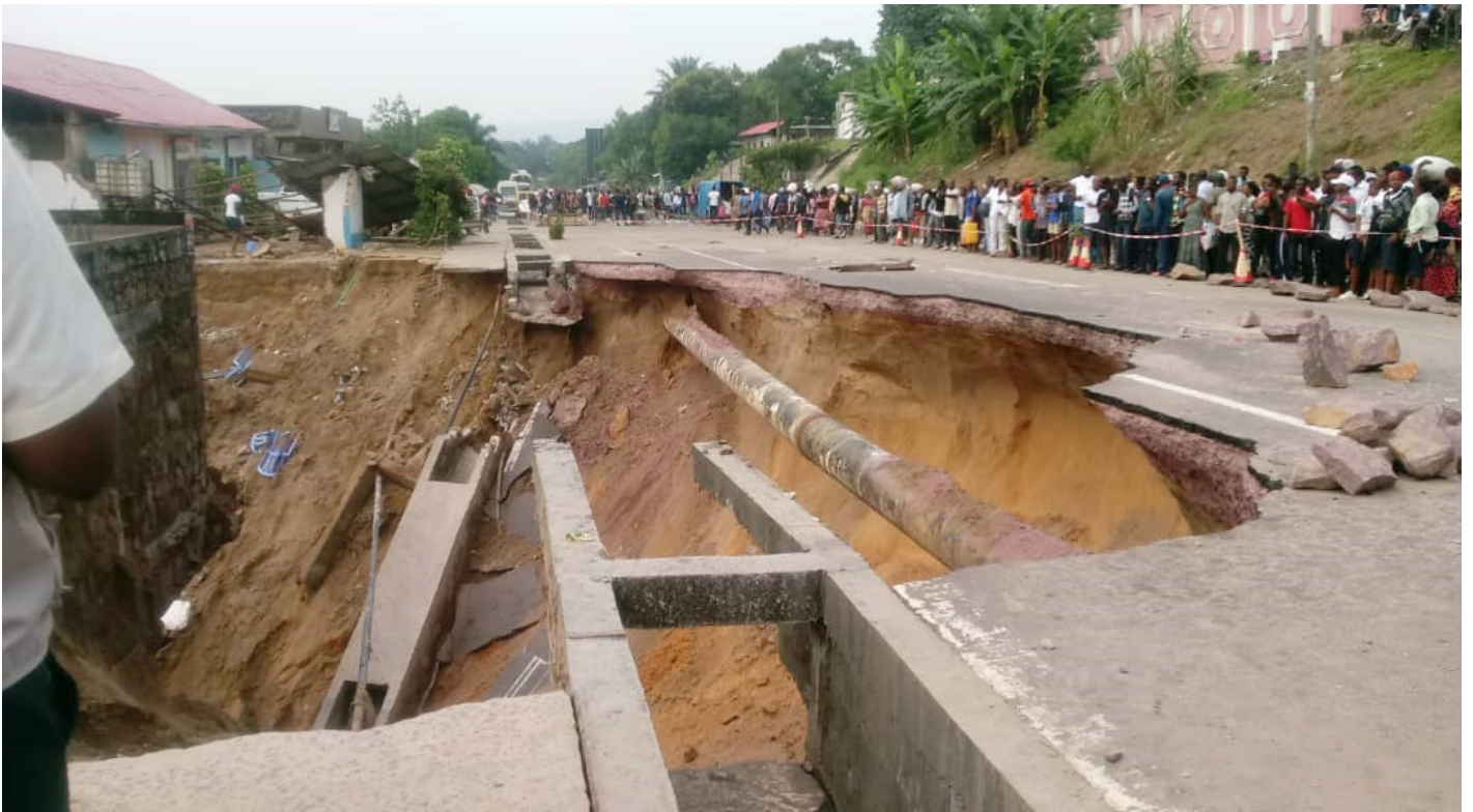
Road erosion during floods, Kinshasa. Jolino Malukisa, 2019.
